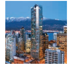
Shangri-La Vancouver Vancouver 2008
