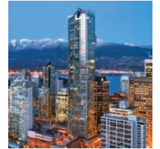
Shangri-La Vancouver Vancouver 2008
